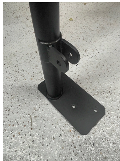
Fork welded to the scuttle brace.
