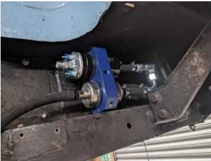
...and in with the new in the rear offside wheel arch—seeing the pump as work in progress. Pipes and wiring still to be installed.
