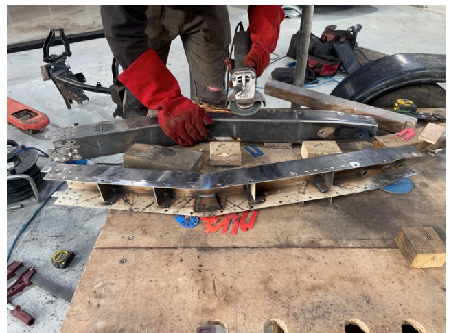
Welding and finishing the chassis legs, showing the Internal strengthening webs
